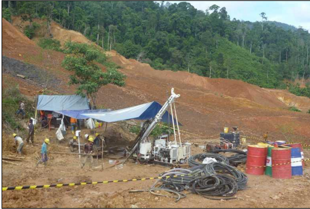
Figure 1: Drill rig set up and ready to commence drilling on hole PNGD020. There is current surface mining activity being undertaken at the site within the Prosperity IUP.
