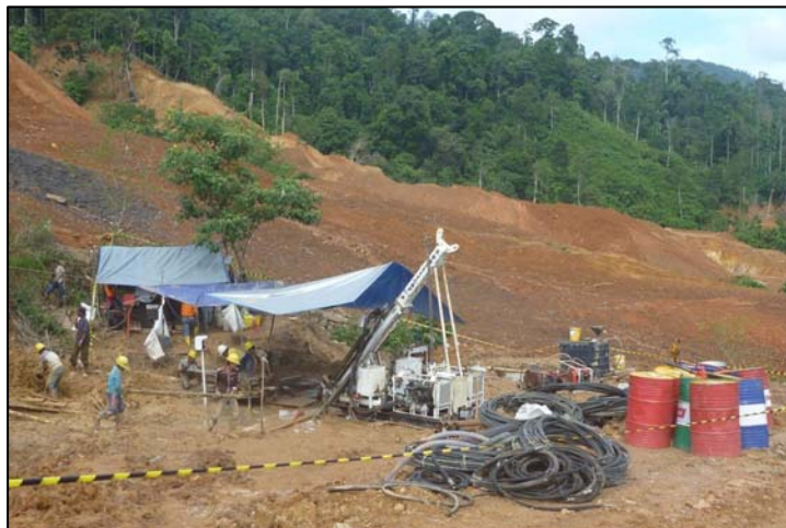
Drilling rig setup at Kuini
